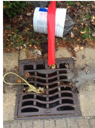
Catch Basin with Pump in Place
